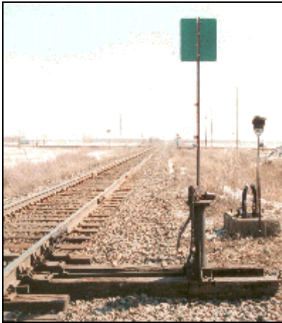
Figure 15 - Switch target for a locked switch. Note lowered position of locked switch handle.
