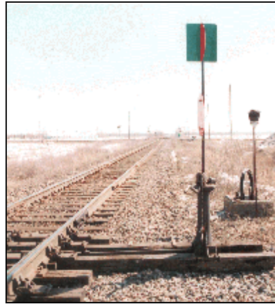
Figure 16 - Switch target for a switch that is slightly open. Note raised position of switch handle on unlocked switch and similarity of target to Figure 15.
