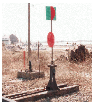
Figure 8 - Typical 31 B switch stand.
