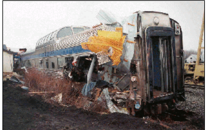
Figure 3 - Damage to Skyline car due to contact with the foundation wall of farm supply building.
