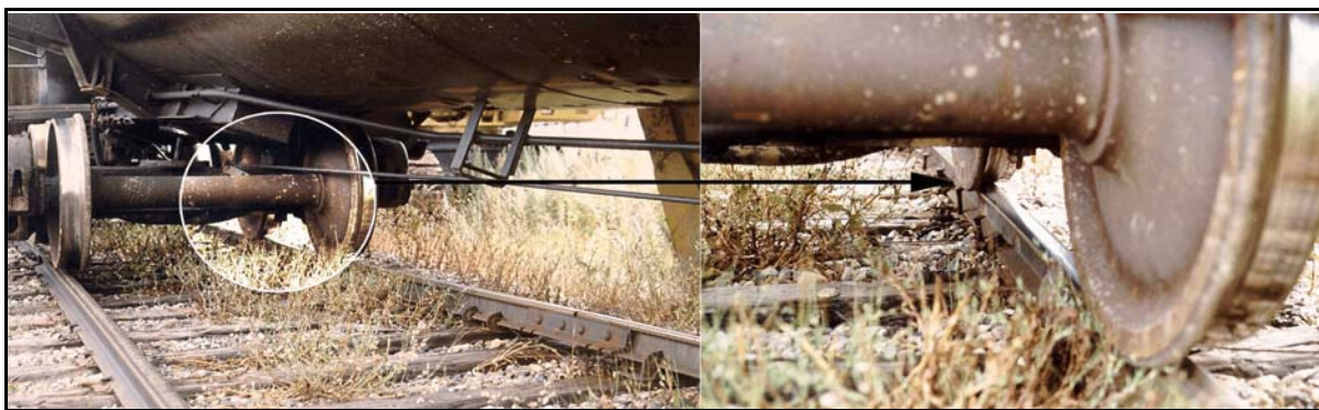
Photo 1. The B-end of car GATX 48058 remained on the canted south rail. A close-up of the shaded area shows the spike lift observed beneath the B-end truck.
