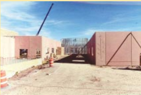
The new Baca Dlo' Ay' Azhi Community School under construction.
