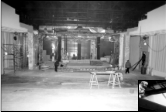
As the work progresses...
