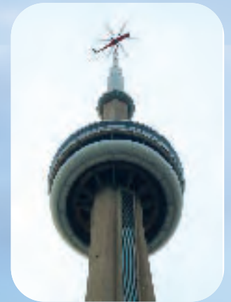
Erickson Aircrane helicopter reenacts antenna topping off of CN Tower for 30th anniversary
