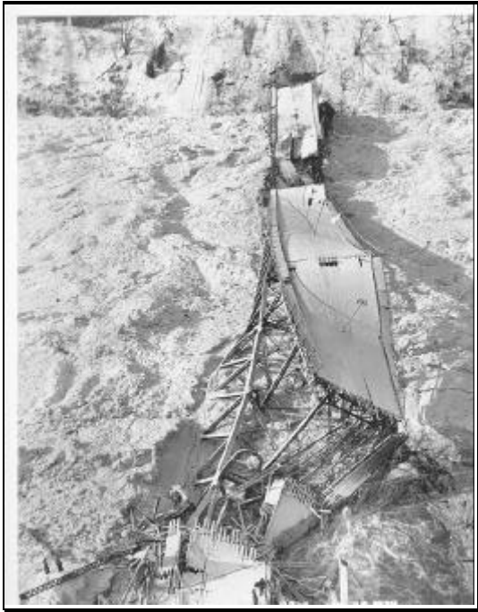
Ice induced collapse of the Honeymoon Bridge - 1938
