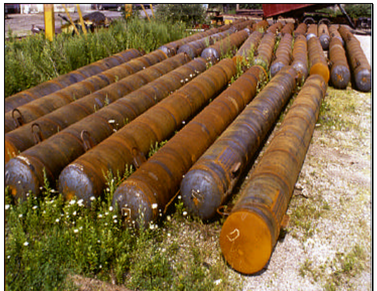
Steel Pontoons that make up the spans
