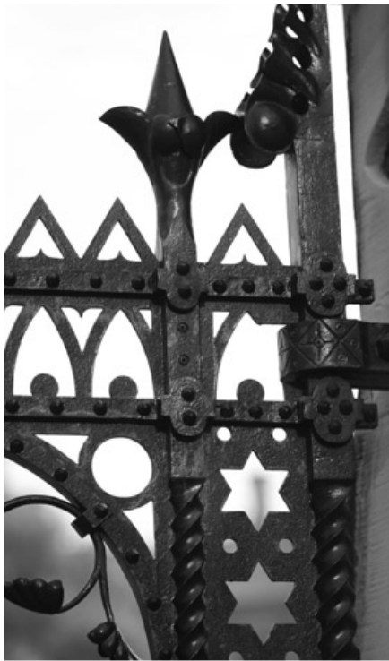
Detail of iron gates, west entrance of Parliament Hill
