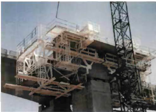
Figure 6 Balanced cantilever – Form traveller
