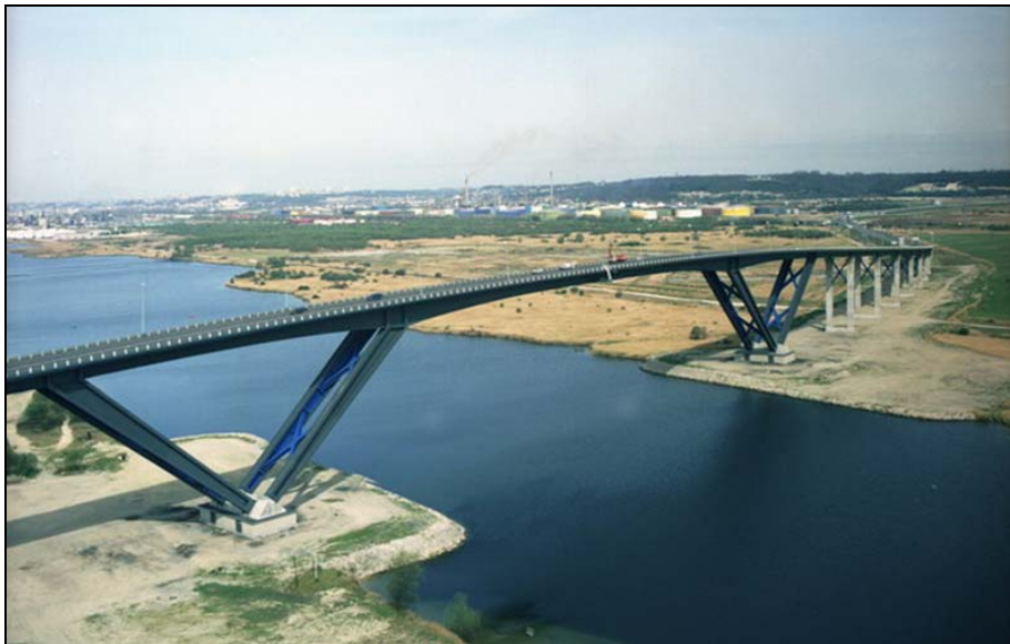
Figure 14 V-shaped piers– Le Havre Grand Canal
