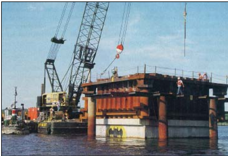
Figure 16 Prefabricated coffer-dam
