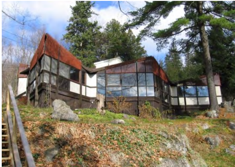
STRUTT HOUSE 1956, AYLMER SECTOR, GATINEAU PARK; SOURCE: NCC
