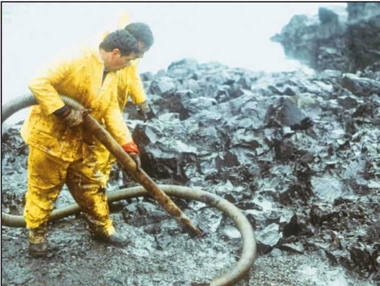
Figure 5.9 Oil Removal by Vacuum Systems
