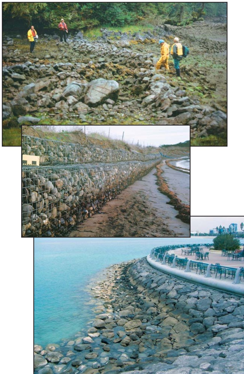
Figure 4.7 Permeable Manmade Shorelines: cobble fish weir archeological site (top photo), gabion baskets (middle photo), and a cobble/boulder seawall (bottom photo)
