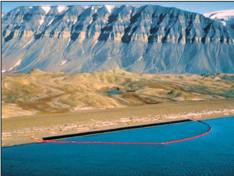
Figure 3.11 Oil is contained on or against the shoreline by use of boom.
