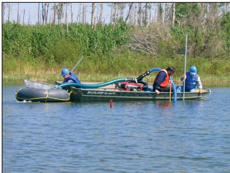
Figure 5.10 Shallow-water Vacuuming of Sunken Oil
