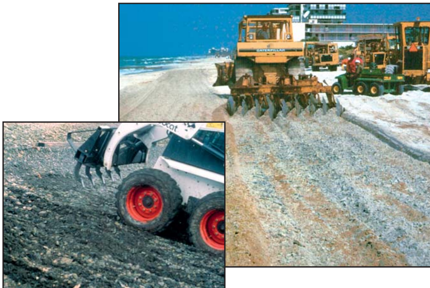
Figure 5.20 Dry Mixing of Oiled Intertidal Sediments on Sand and Mixed Sediment Beaches
