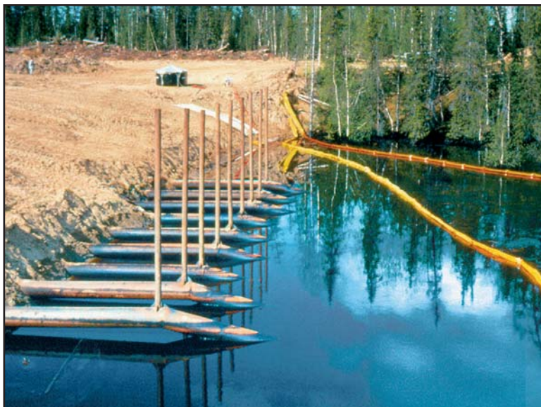
Figure 3.19 Earth Dam with Multiple Siphon Pipes
