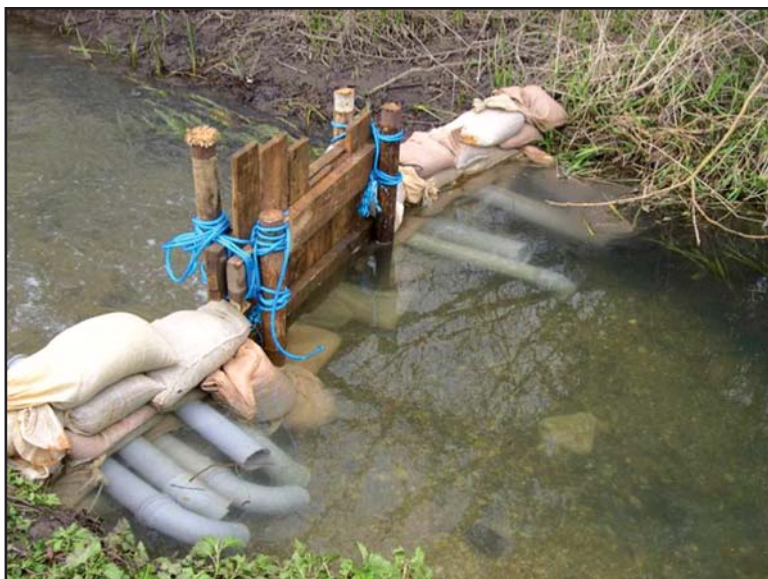
Figure 3.20 Channel Barrier – Sand Bags, Wood, and Underflow Pipes
