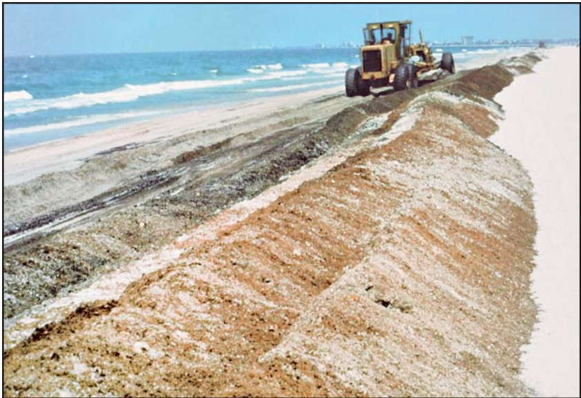
Figure 5.15 Two-stage Removal with Grader Supported by Front-end Loader or Elevating Scraper
