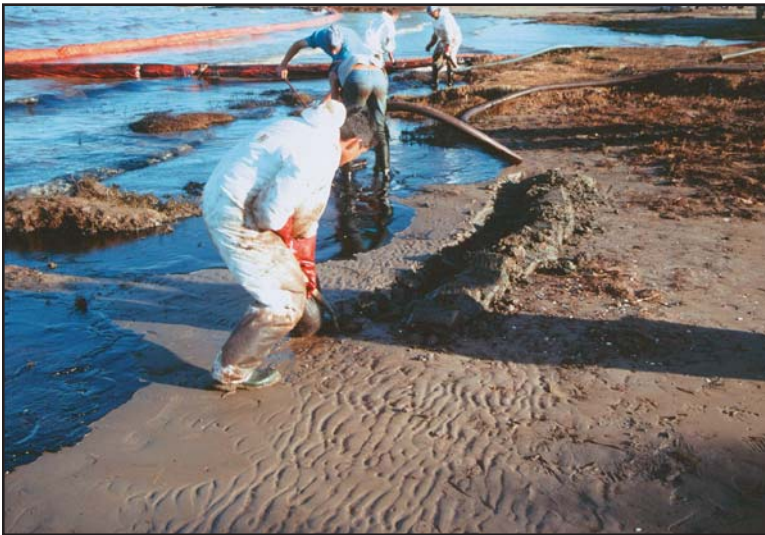
Figure 3.13 Digging a Collection Trench on a Sand Beach
