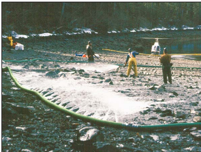
Figure 5.3 Flooding with perforated header hose on the upper beach.
