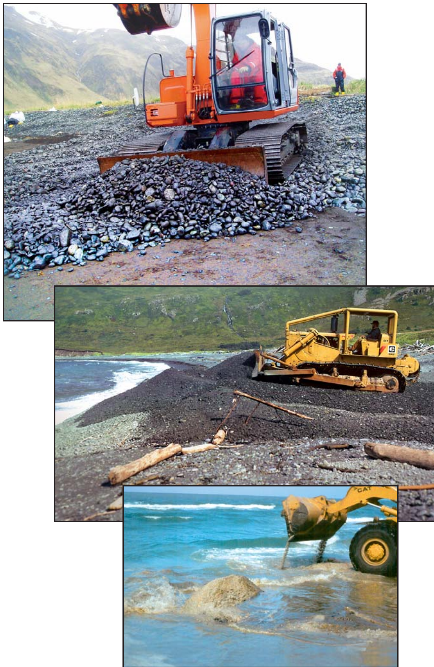
Figure 5.22 Oiled sediment is relocated from the upper to the lower intertidal zone where there is a greater potential for sediment reworking.
