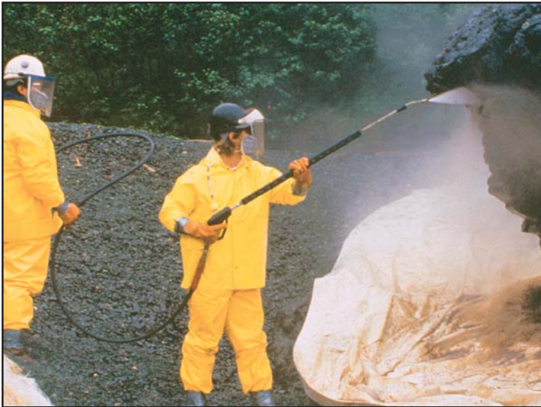
Figure 5.6 High Pressure Washing
