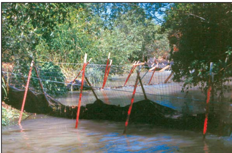
Figure 3.17 Channel Barrier – Silt Screens
