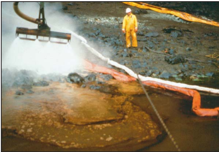
Figure 5.5 Low-pressure Warm Water Washing
