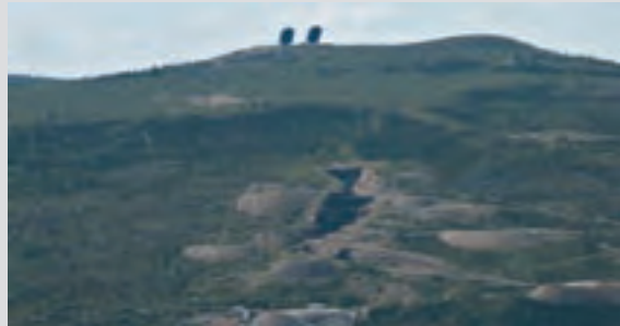
The billboard antennae on top of Galena Hill, a highly visible local landmark, were used for communications between the south and the defense systems based in the arctic. Below the towers, the slot-like hole of the Mackeno Mine is a late 1960s open pit along the vein. Peter Long
