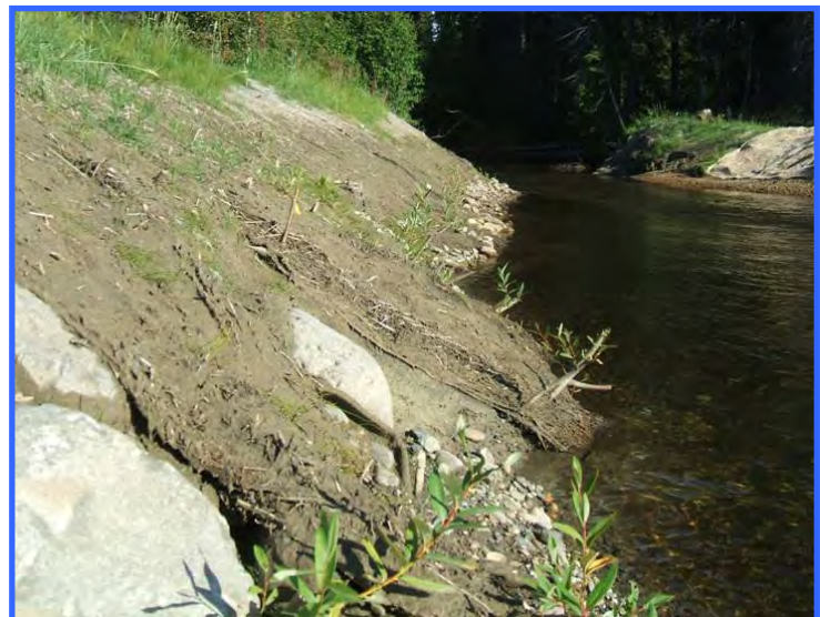
The same site as above one year later. Grass is emerging and the willow cuttings are growing along the water. The slope may look exposed and prone to erosion, but the buried matting is keeping the slope stable while vegetation becomes established.
