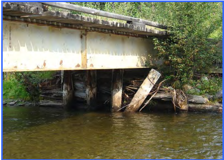
The abutment and approach (not shown) of this bridge failed because surface drainage water flowed to the bridge rather than being directed away from it. This could easily have been prevented with proper grading and bridge design.
