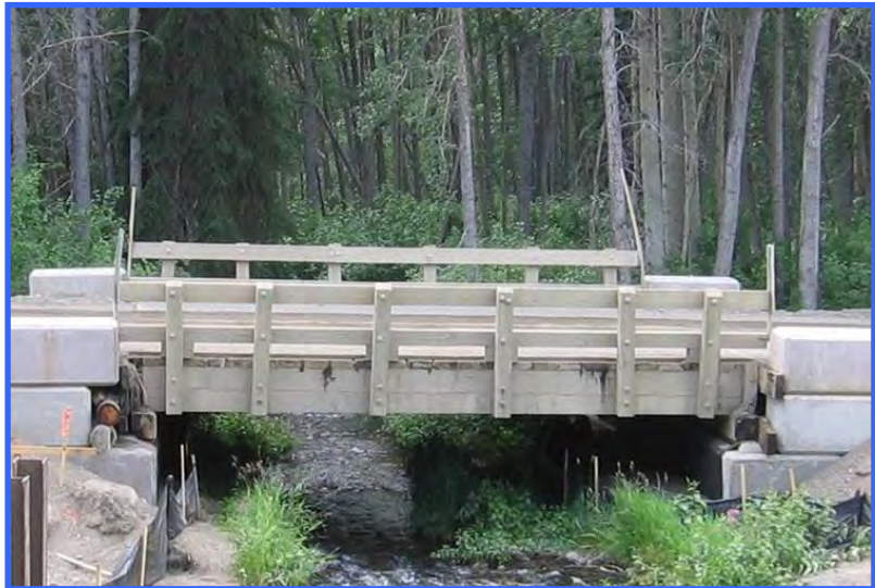
A properly-installed temporary clear-span bridge with perimeter silt fences.
