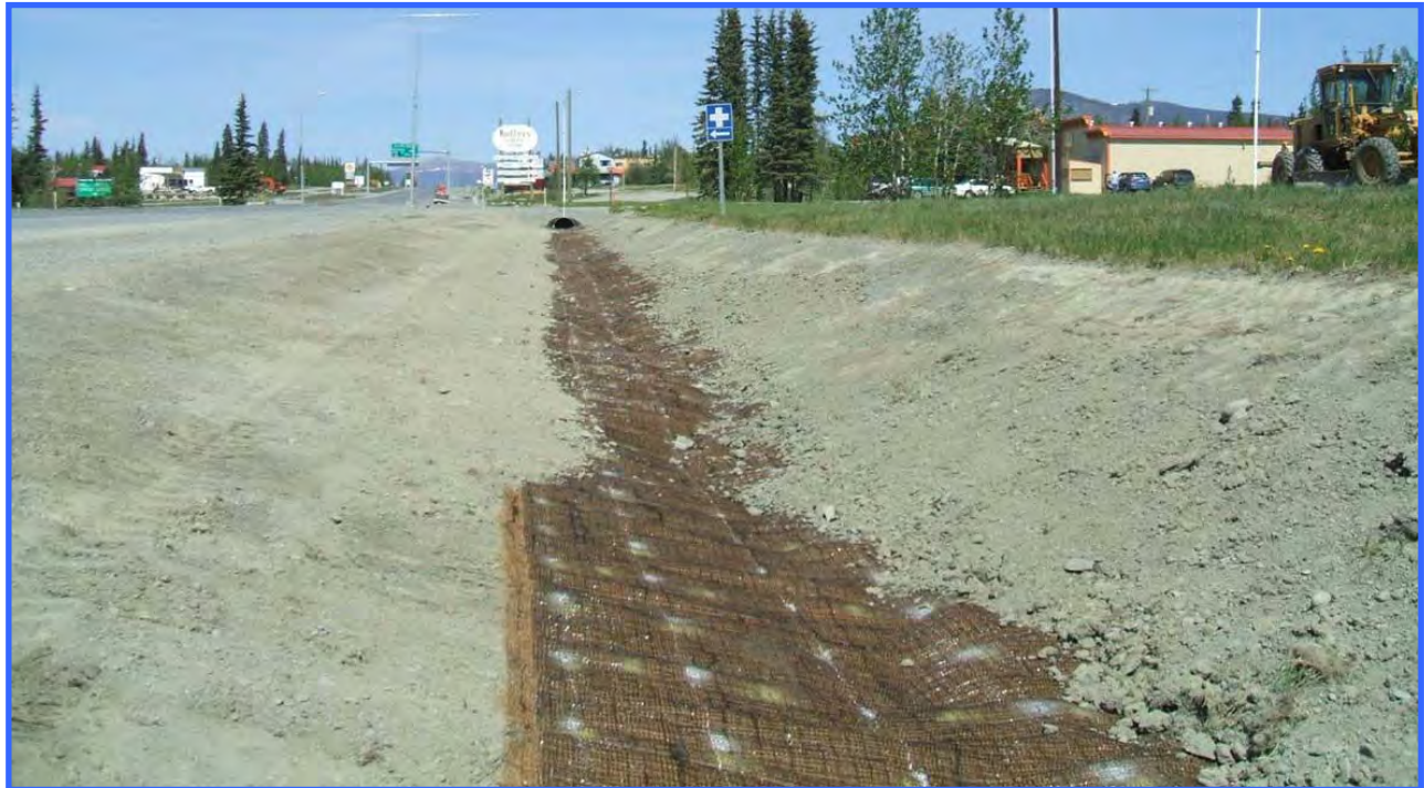
Coconut fibre matting reinforced with a UV resistant mesh was installed in this erosion-prone ditch that drained directly into an adjacent river. The site was seeded prior to installation of the matting. There are two installation errors to note: the edges of the matting should have been folded into the side slopes by means of an anchor trench, rather than lying flat on the ground. Also no dirt should have been put on top of the matting.
