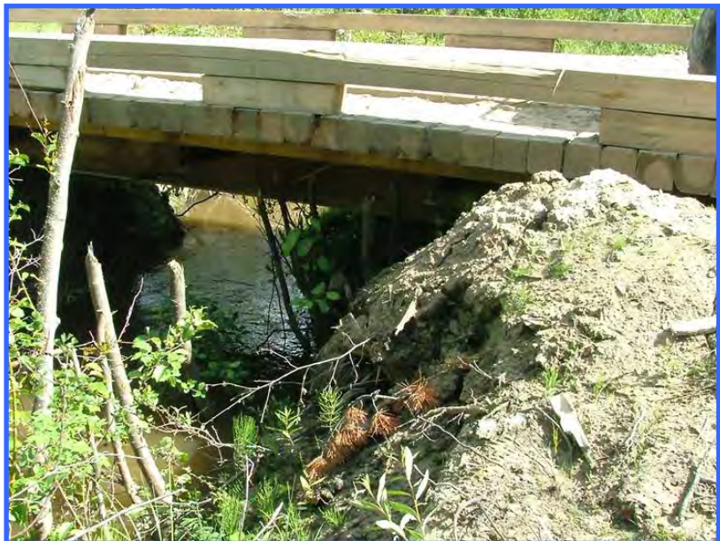
The abutment of this clear-span bridge should have been protected with riprap. Embankment collapse and sediment release are imminent.
