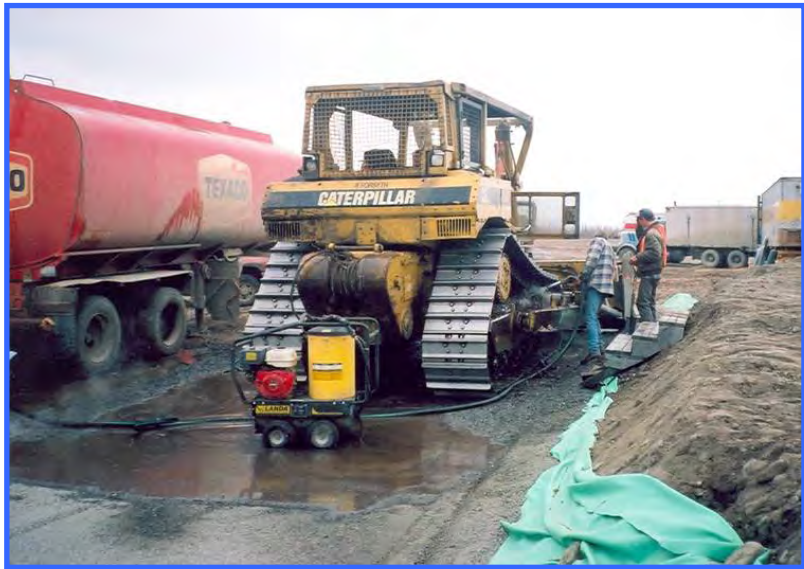
Pressure washing a dozer in a designated site that was lined and bermed.
