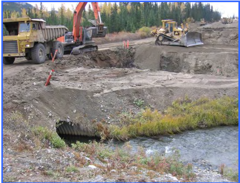
The site of a new culvert crossing is being prepared “in the dry”, while the stream is left undisturbed. The old culvert and channel will be reclaimed after the new one is activated.
