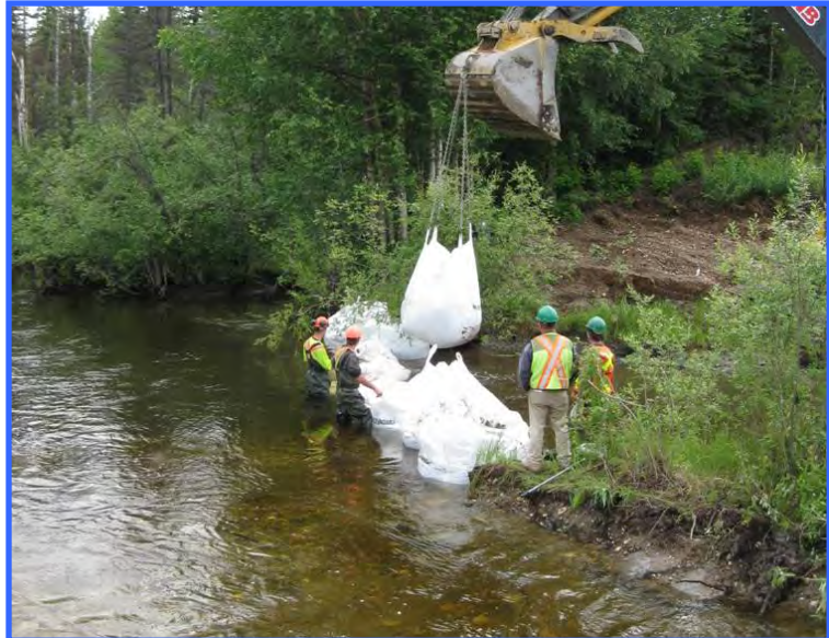
The same site as above. Watson Creek is being blocked off with large sand bags and the flow is captured by the diversion channel (foreground).
