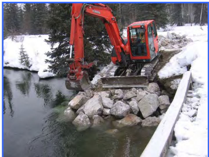
A temporary ramp consisting of large, clean rock infill was constructed so the excavator could access the stream and work underneath the bridge. After the work was completed, the rock was removed.
