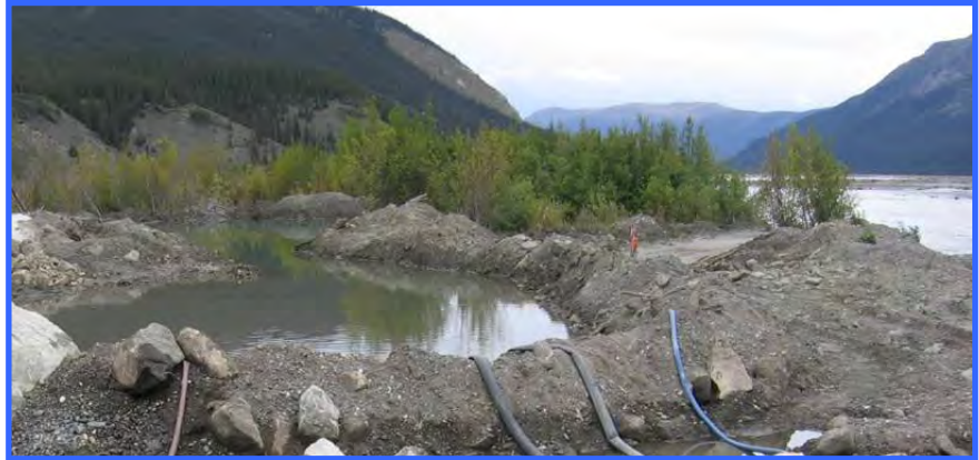
This sediment trap contains water pumped from isolated in-stream work areas created to construct a new bridge pier. This sediment trap has a passive overflow so clear water can exit the overflow and pass through vegetation before re-entering the adjacent stream.
