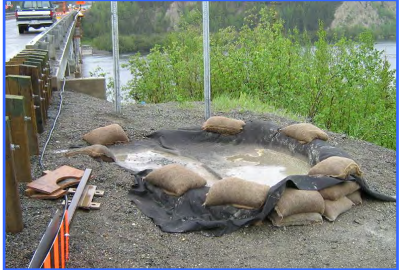
The size of a sediment trap depends on the volume of water that will be generated and sediment settling rate. This trap, while small, was built to contain a small volume of concrete curing water, and was adequate for the job.
