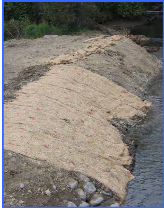
A manufactured erosion control product composed of straw and jute mats being installed along a creek. The surface was seeded before the matting was unrolled, and willow cuttings were later planted at the water's edge.
