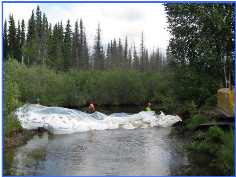
The same site as above. The sand bags are covered with plastic on the upstream side of the diversion. The plastic is anchored on the bottom with rocks to hold it in place and to seal the stream blockage.
