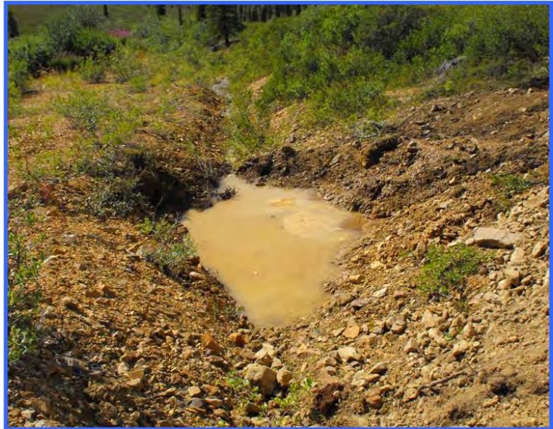
A small excavated sump built to collect runoff from a drill site. This is a simple but effective method for reducing sedimentation.
