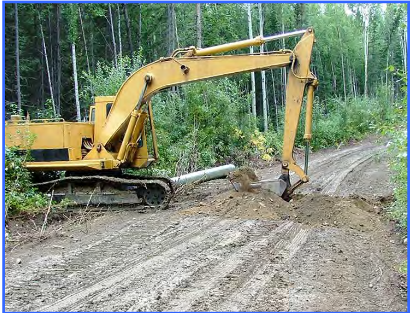
Installation of a culvert to provide cross drainage.
