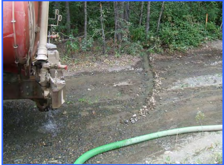
A simple diversion was created to guide runoff into the vegetation, rather than the stream. Sometimes it's the little things that make a big difference.
