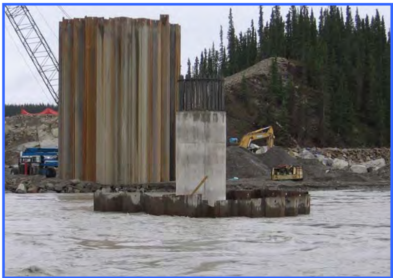
Cofferdams used in construction of bridge piers.
