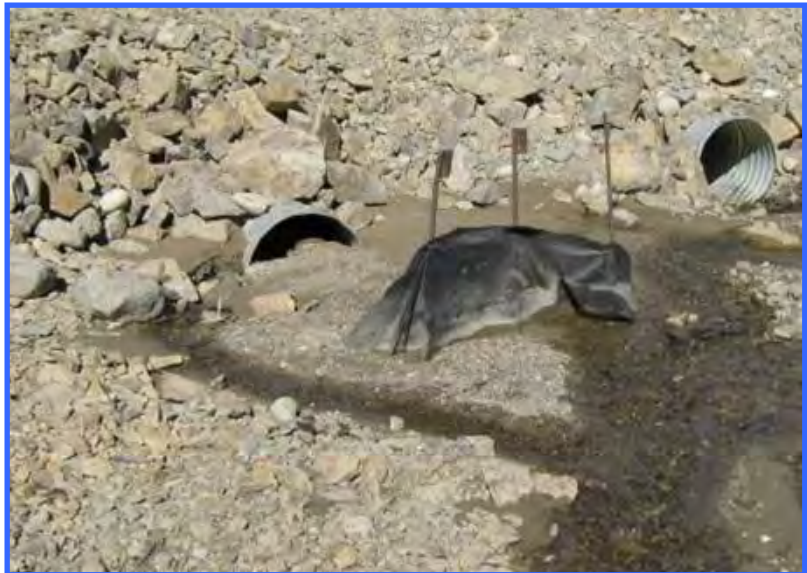
The attempt to keep this culvert (on left) from filling with sediment was too little and too late (the culvert on the right is only intended to be a high water overflow pipe). The silt fence is inadequate for the size and amount of sediment, and for high water flow velocities. The problem with two pipe systems is that the lower one fills with sediment during high water events if there is a lot of sediment flowing through the creek, such as this one. A much larger culvert should have been installed to avoid this situation.
