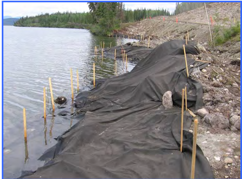
All that was available on short notice for use as a temporary erosion control measure on this road building project was unwoven geotextile cloth. While not the preferred material, this impromptu action on the part of the contractor was a resourceful solution, and was well-executed (note the ample staking). A week later, the permanent solution was installed and consisted of large rock (riprap) placed along the bank.
