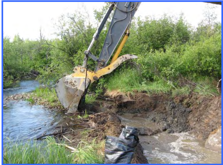
The same site as above. The downstream earth plug is being removed.
