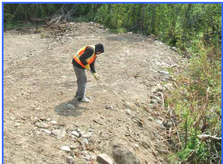
A small area next to a creek is raked in preparation for seed application.
