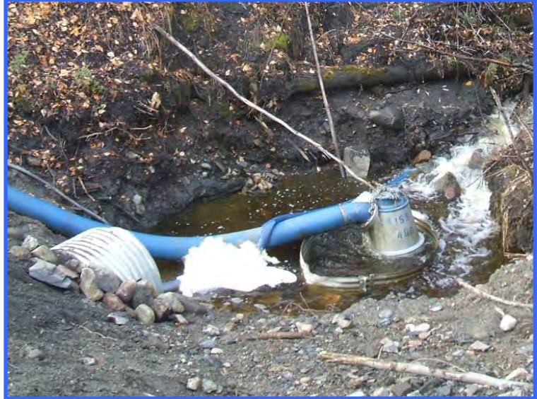
A pumped diversion showing the water intake. Even for this small stream, pumping its entire flow across the work site required large volume pumps.
