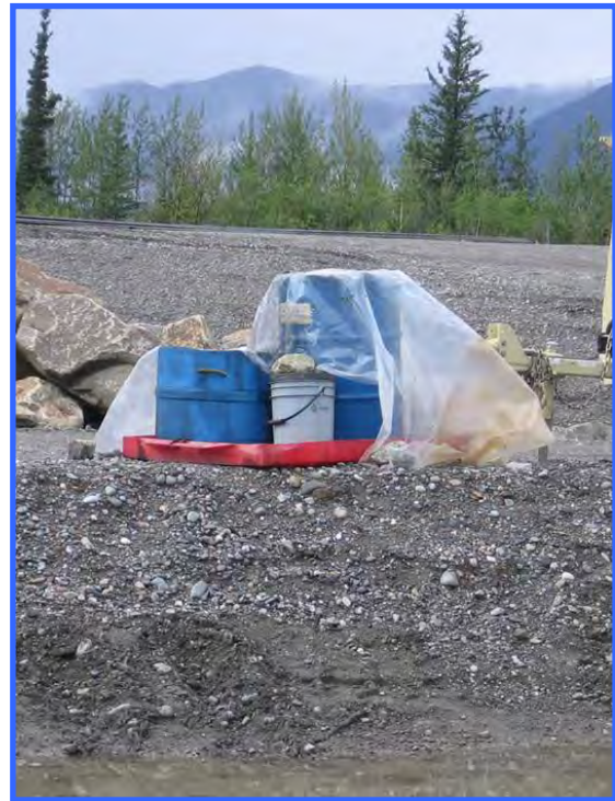
While these drums of fuel and lubricants were placed in a spill tray and an attempt was made to cover them, the protection is not adequate. The plastic half drum and spill tray will collect rain water. Workers will be tempted to tip the containers to dump out the water and the lighter petroleum products will be the first to overflow. Note also that they are not stored 30 m away from the water body in the foreground.
