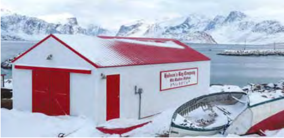
Hudson's Bay Company interpretive and restoration building work completed to date.
