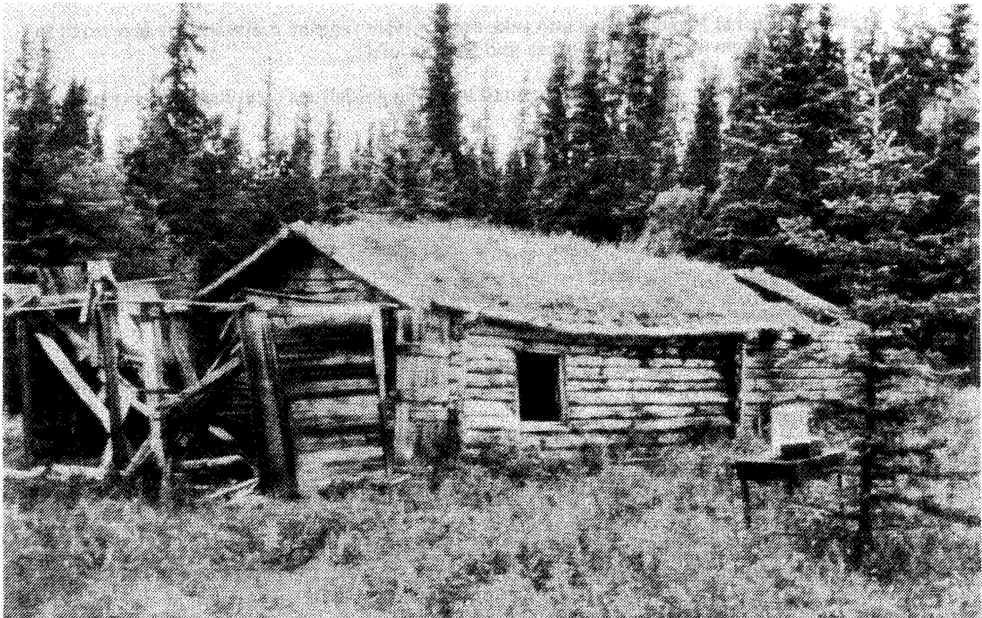
The top photo shows Ship Yard Island with the remains of the steamer, Evelen/Norcom. The lower photo shows a sod roofed cabin at 17 Mile Wood Camp. Note collapsed roof section at rear.
