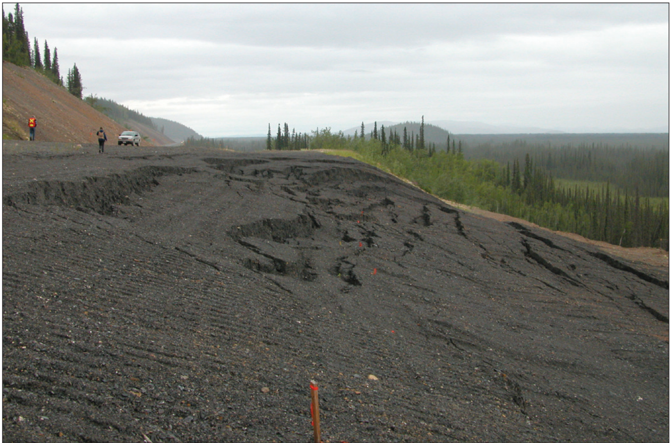
Subsidence of road fill along the Alaska Highway near Beaver Creek caused by permafrost thaw beneath fill. The failure is not directly linked to climate change — rather it was caused by disturbance of groundwater flow pathways which has led to permafrost thaw at this site. But it is representative of the type of failures that could occur along highways as permafrost starts to thaw more.
