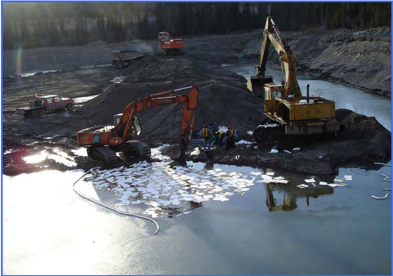
An emergency response situation. An oil spill occurred on this small lake during gravel extraction activities when a crack developed in the oil reservoir of an excavator. Booms are being deployed to contain the spill, and oil on the surface is skimmed off using absorbent pads. Ice on the lake helped contain the spill.
