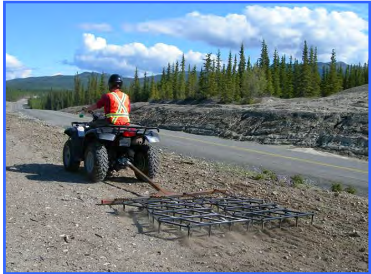
A harrow is used to loosen the surface soil prior to seeding. Seeding projects can often be completed by a two-person crew using an ATV equipped with a harrow and broadcast seeding, in conjunction with hand seeding.
