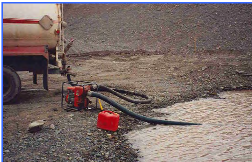
An unacceptable pump station. Water pumps need to be placed in spill trays and fuel must be stored >30 m away from any water body.
