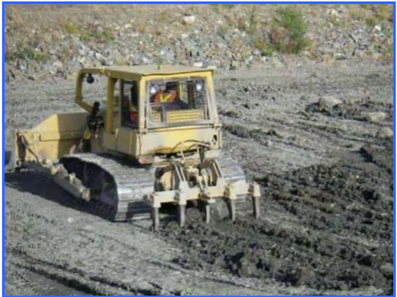
Extreme roughening of the soil surface using a ripper.
