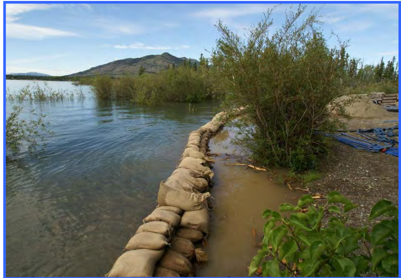
Sand bags being used to protect an eroding lake shore. Note the clear water in the lake and the turbid water along the shore.
