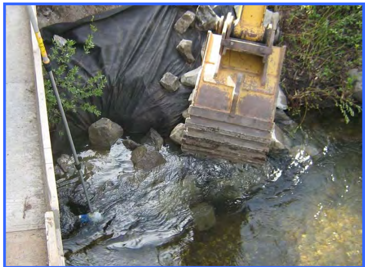
Careful placement of clean rock along a stream bank. A water sample is being collected to measure the turbidity caused by sediment release.
