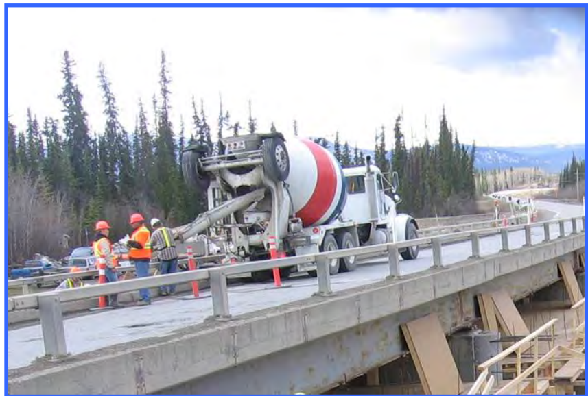
A sturdy work platform constructed below this bridge allowed easy access to the superstructure, but it also helped catch debris and keep uncured concrete from falling in the water.
