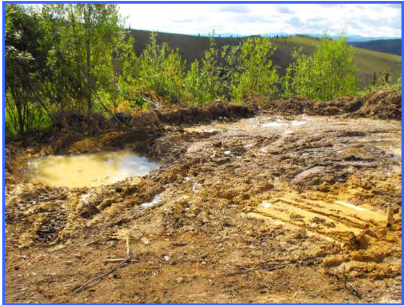
Decommissioning of this drilling pad is nearly complete. The sump is left and the site still needs to be reclaimed. Note the pile of organic material piled along the edge of the vegetation. This will be spread over the mineral soil and the site will be seeded.
