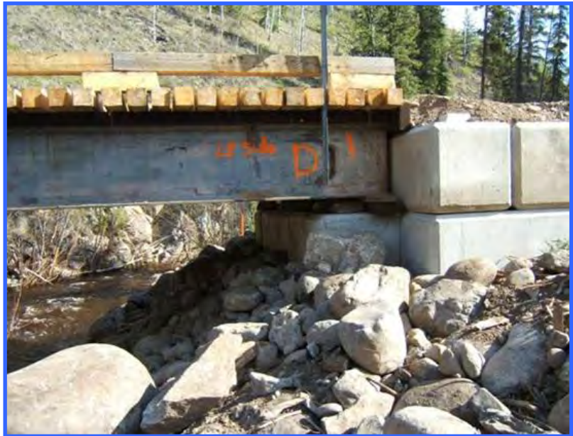
A properly-installed permanent clear-span bridge with riprap for bank protection.
