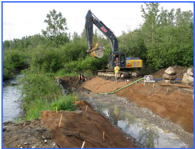
The project in this photo and the following photos involved lengthening two existing culverts at Watson Creek. To complete the work, the creek had to be diverted so the culvert extensions could be completed in the dry. This photograph shows the diversion channel on the right and Watson Creek on the left. The banks are lined with jute fabric to protect them from erosion. The new channel is being washed and the sediment-loaded water is being pumped out into the vegetation.
