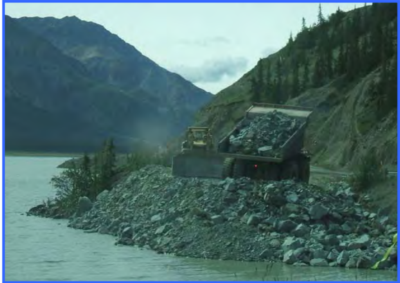
For this road-widening project, the lake edge had to be infilled. The procedure involved dumping rock on the ramp and then carefully push it into the lake with a dozer.
