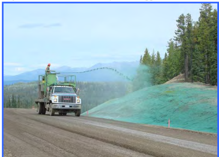
Hydroseeding in progress. A slurry containing fibrous mulch, seed and fertilizer is sprayed onto the slope to reduce erosion potential and promote quick revegetation. A tackifier is often included to hold the mixture together.
