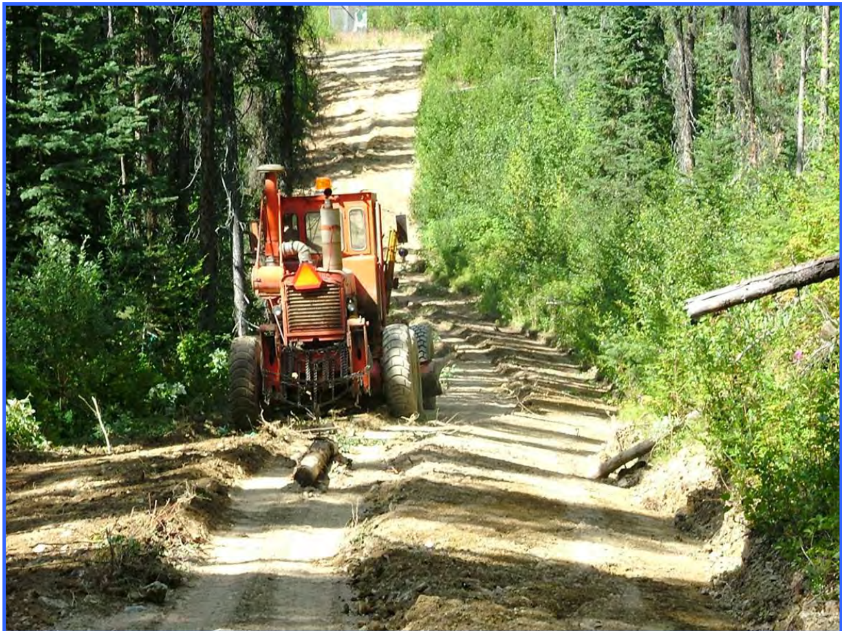
Proper sloping, crowning, and ditch placement on this road is creating good drainage and a stable roadbed.
