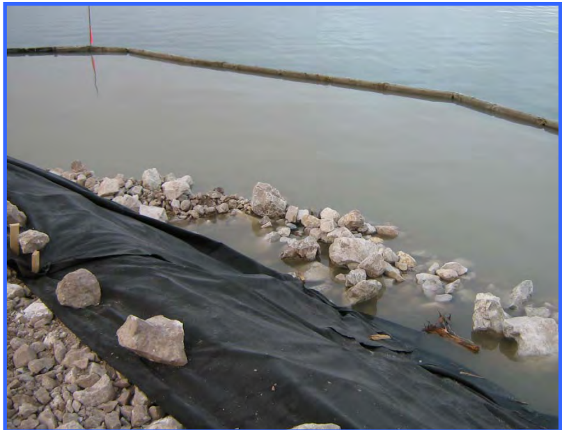
Little Atlin Lake boat ramp is being expanded. Infill area in the lake has been isolated with a silt curtain to contain sediment. Note the turbid water inside of the silt curtain compared to the clear water beyond.
