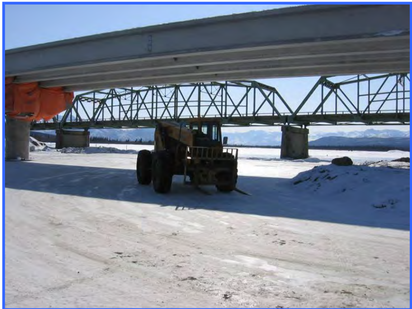
Working from the ice is often the best way to access the underside of bridges, and makes it much easier to protect water bodies. In this case, an ice bridge across the Donjek River was built to facilitate construction of a new bridge.
