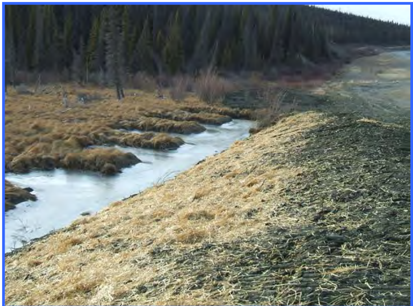
Straw mulch used to protect a seeded stream bank from erosion. This straw should have been worked into the ground surface better so it will not blow away or wash into the water body.
