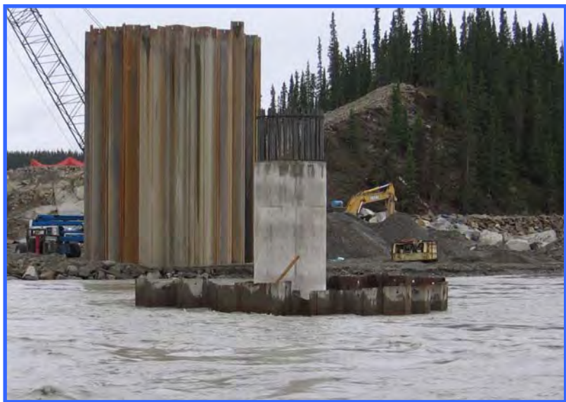
Cofferdams used in construction of bridge piers.
