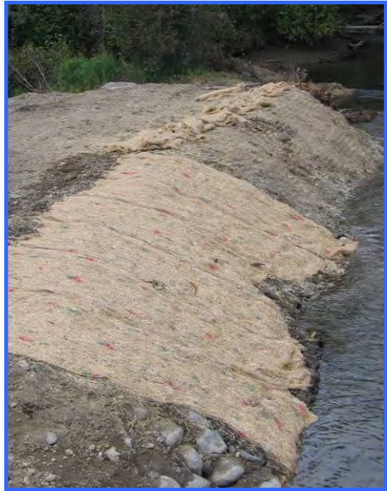
A manufactured erosion control product composed of straw and jute mats being installed along a creek. The surface was seeded before the matting was unrolled, and willow cuttings were later planted at the water's edge.
