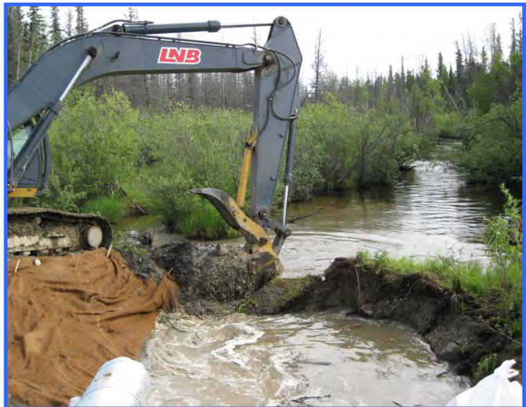
The same site as above. The upstream earth plug is being removed.
