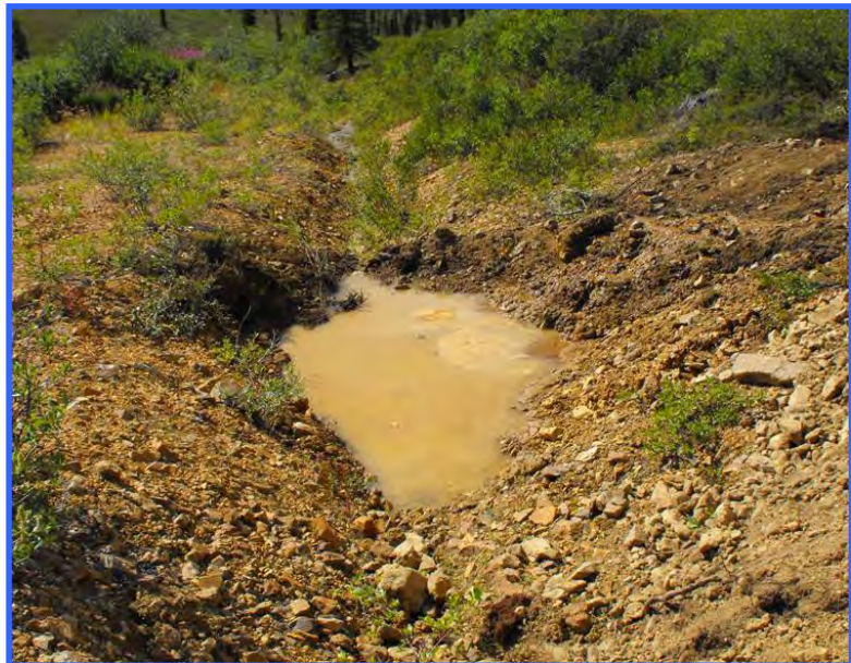
A small excavated sump built to collect runoff from a drill site. This is a simple but effective method for reducing sedimentation.
