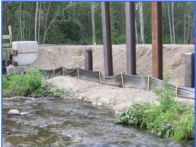
This silt fence was installed along a creek as a perimeter fence to keep loose material from rolling into the water.
