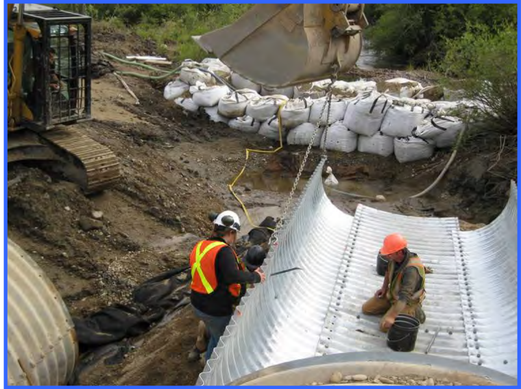
The same site as above. The work area is dry and the culvert extensions are being attached.
