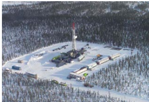
Well site K-58 completed by Devon Canada Corporation in Eagle Plain. Photo taken March 14, 2005. (Marc Dionne, Client Services & Inspections Branch)
