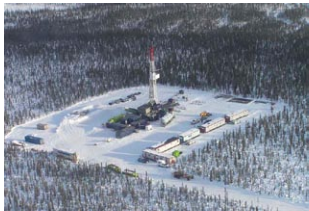
Well site K-58 completed by Devon Canada Corporation in Eagle Plain. Photo taken March 14, 2005. (Marc Dionne, Client Services & Inspections Branch)
