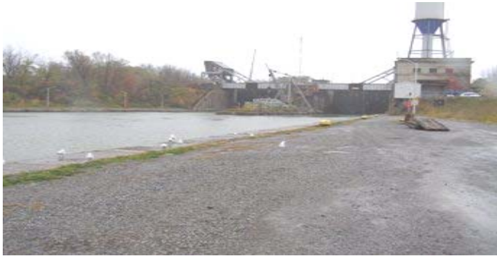
Photo 3. Lock 4, looking upbound (towards Lock 5)
