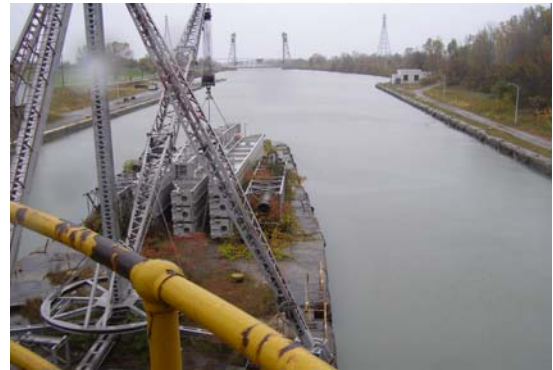
Photo 4. Bullnose, looking downbound towards Lock 3
