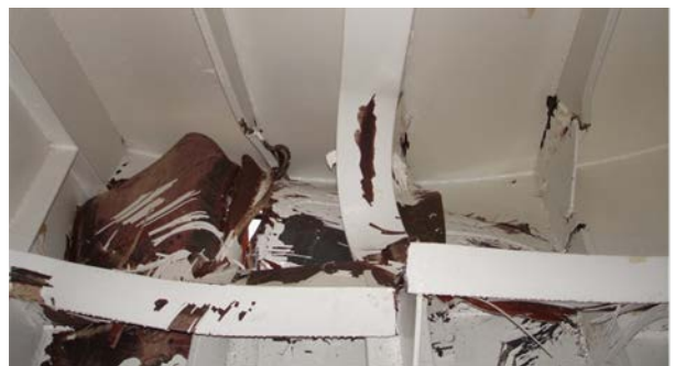
Photo 3. Interior damage to bow visor
