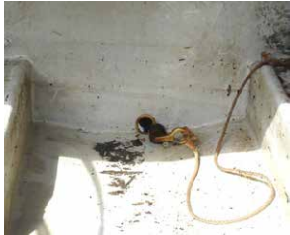
Photo 2. Drain hole and removable plug
