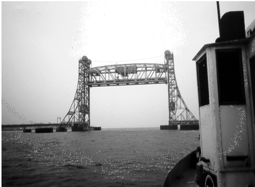
THE SAINT-LOUIS BRIDGE IN THE UP POSITION
