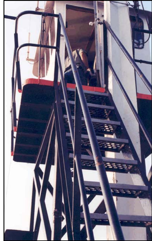
Photo 3. Stairway to upper wheelhouse
