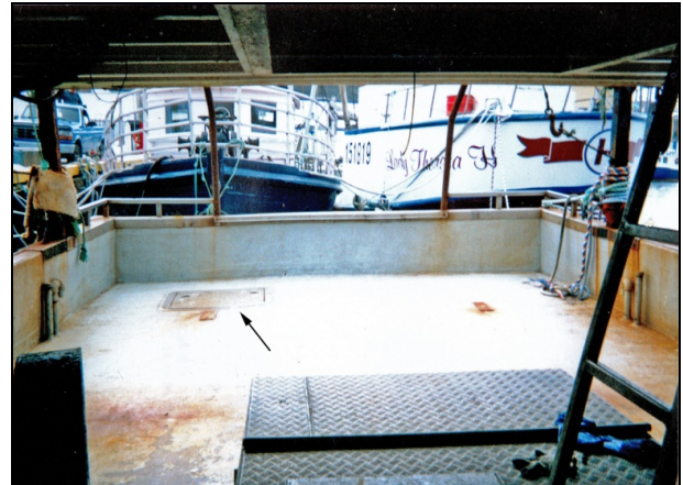
Photo 2. Access hatch to lazarette.
