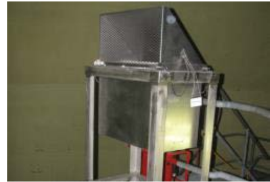
Hydrogen Control and Mitigation with licensees have enhanced hydrogen control through installation of Passive Autocatalytic Recombiners.
