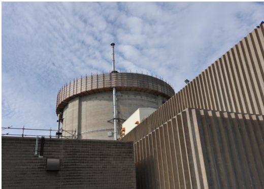
Point Lepreau Emergency filtered vent stack
