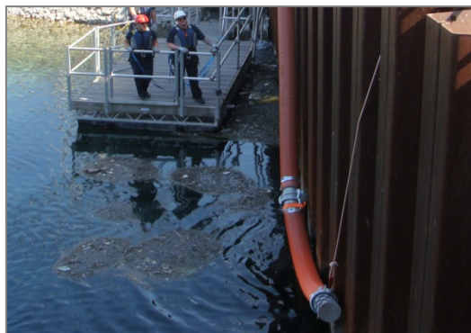
Darlington Emergency water supply.
