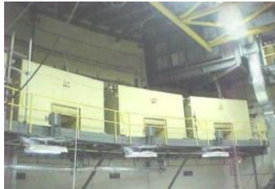
Containment cooling enhancement to SAMG or through repowering Containment Air Coolers (plant specific approach based on design)
