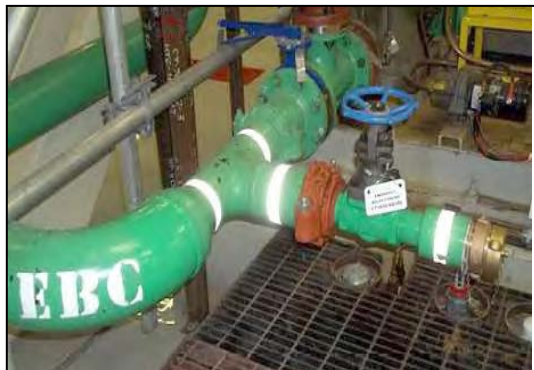
Water Supply Connection Points
