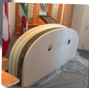
Remodeling the new Chamber
