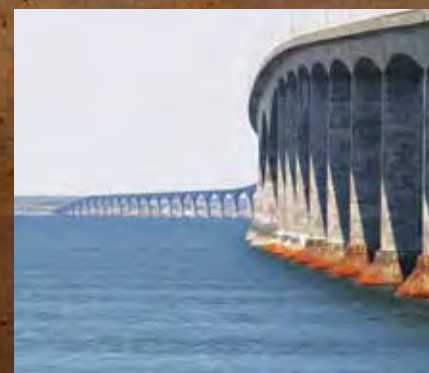
Confederation Bridge, looking toward PEI
