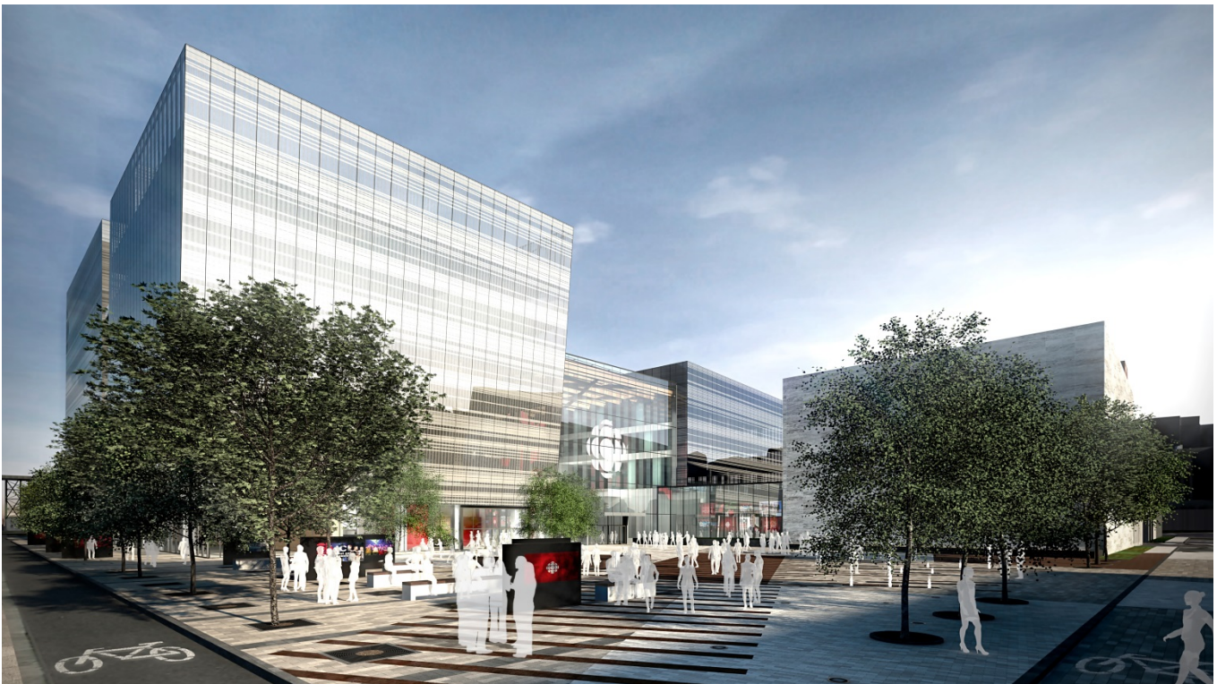
Work on the new Maison de Radio-Canada is getting underway and gradually taking shape.
