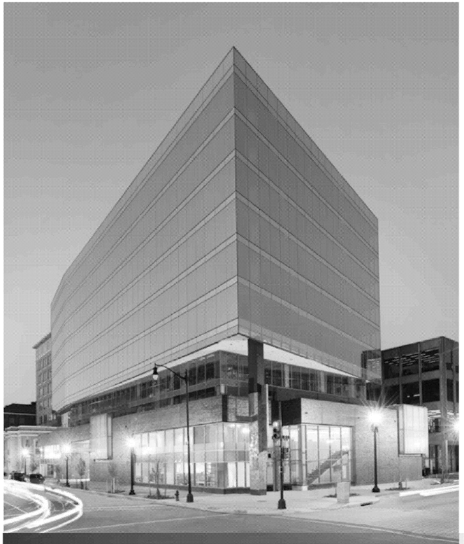
The ability to knock out panels on every floor so tenants could install internal stairs was an important part of Skanska USA's significant structural redesign of 733 10th Street in Washington, D.C.
