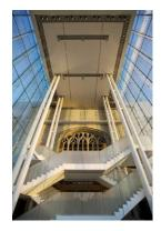
**Innovative Engineering Solution:** Unlike David Ewart's original heavy tower, the new structure does not impose any weight on the existing masonry walls. The Queens' Lantern actually hangs from a specially constructed roof that is cantilevered from concrete walls for the new elevator shafts inside the building. Four large steel columns provide the structural support for the roof, from which hang the panes of glass that form a transparent box.
