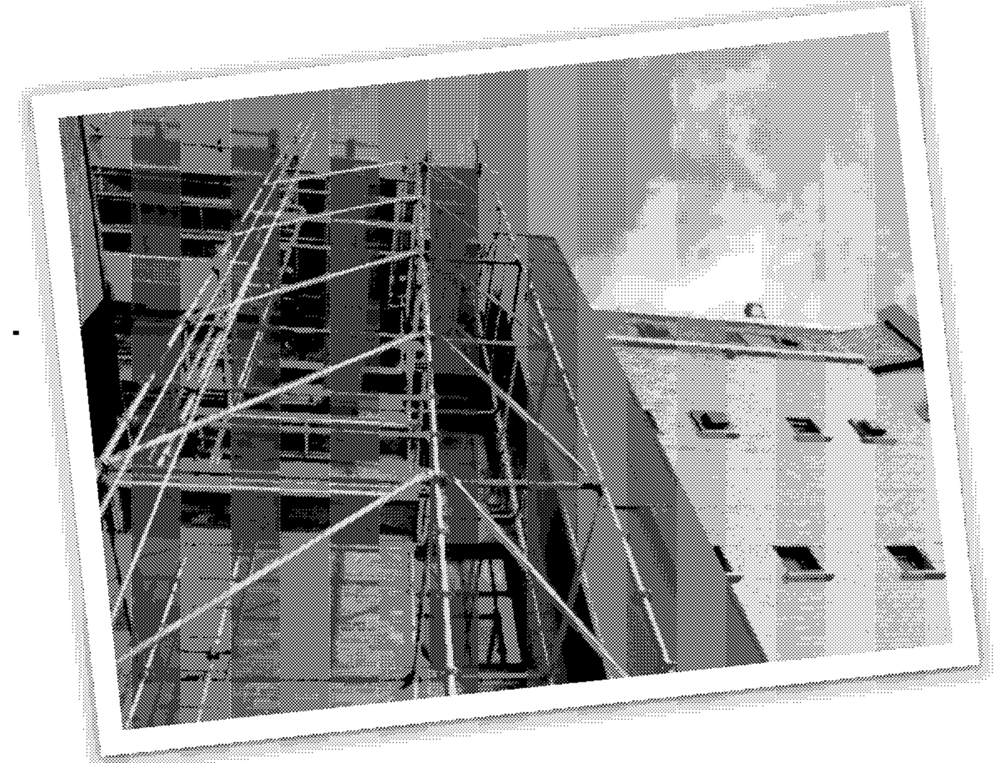
Scaffolding and brick-netting has been put in place permanently to mitigate deterioration that is evident in both locations
