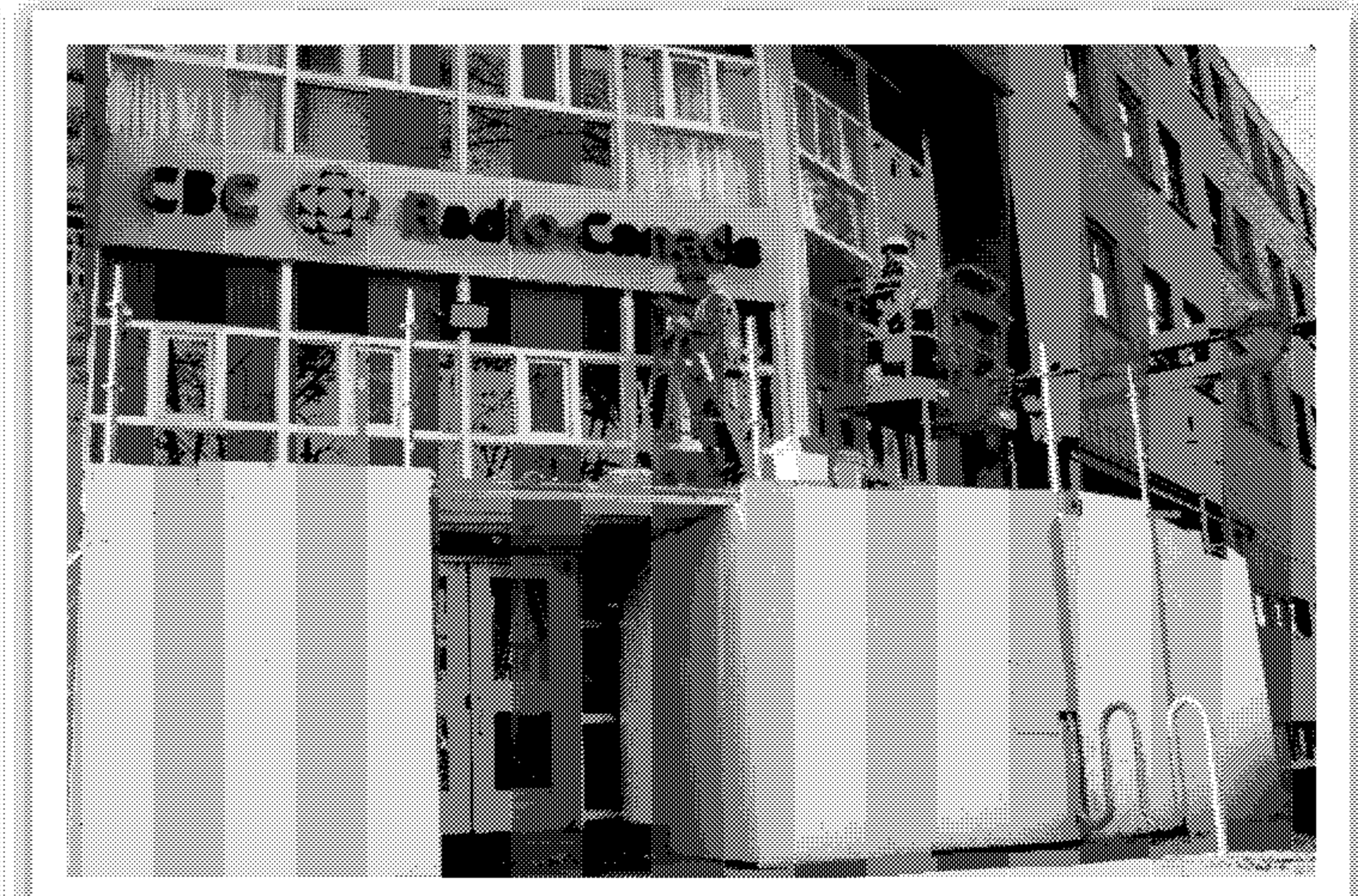
Scaffolding and brick-netting has been put in place permanently to mitigate deterioration that is evident in both locations
