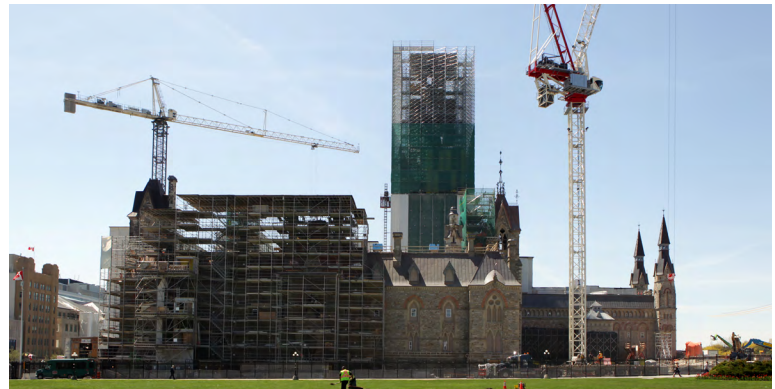
West Block restoration
