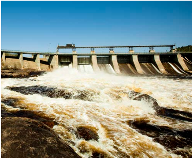
Hydro Dam in Saint-Maurice, Quebec
