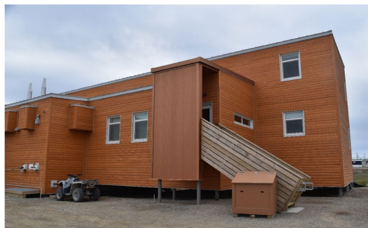
Figure 1: Triplex residence at the Canadian High Arctic Research Station (CHARS), where the greywater system will be installed in November 2018.
