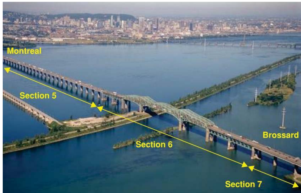
Figure A9 General View of Champlain Bridge
