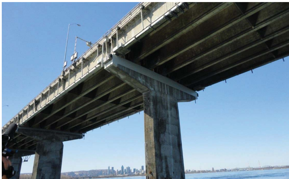
Figure A11 Typical Concrete Span in Section 5 & 7
